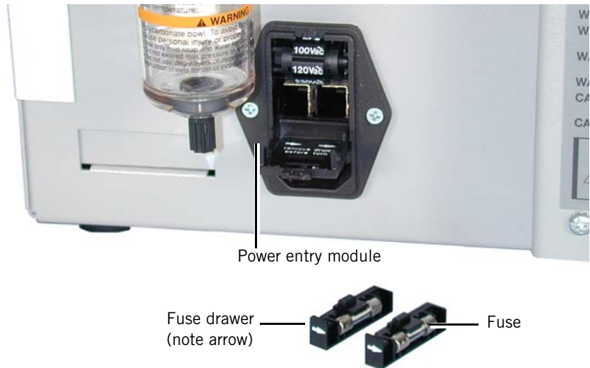
Figure 5-8: Replacing the Fuses
