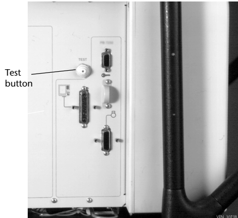
Figure 3-1. Test button location
